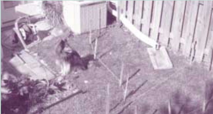
Twine and stakes used to lay-out area for rain garden
