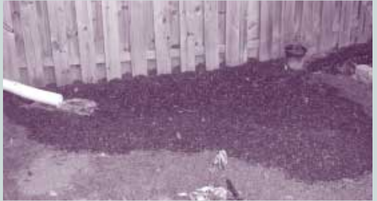
Same rain garden immediately after excavation and soil amendments and mulch added, prior to planting
